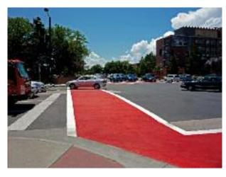
T-28 is an acrylic-based resin system used for pavement area markings and anti-skid surfacing. T-28 is typically used for demarcation of bicycle and pedestrian paths, bus stops/lanes and other specially designated areas.
