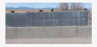
Transpo installed 100 LF of **Screen-Safe™** as part of a test performance. Albuquerque, NM was experiencing problems with the existing material: The barrier's blades cracked at the foundation and blew away from the strong winds in the area. The New Mexico DOT decided to replace a part of the existing material with **Screen-Safe™** to see how Transpo's product fared in adverse conditions.
